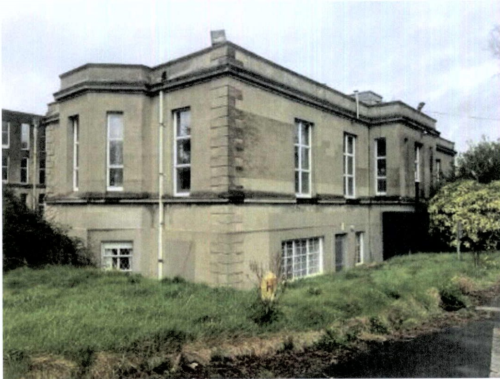
Plate 47: Finlay Wing from new Sandford Road entrance, rendered finish with raised quoins
